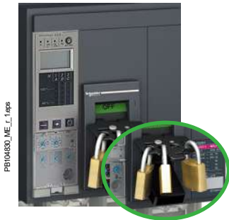
Toggle locked by removable padlocking device.
