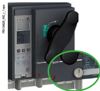
Rotary handle locked by a keylock.
